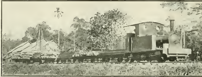
WORK TRAIN IN BRITISH NORTH BORNEO.
